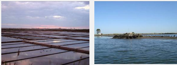
Figure 8 | Left: saltpans habitat for waders; Right: collapsed saltpans (© A.I. Lillebø).
